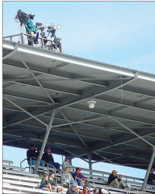
Figure 2.103 High atop a racetrack's grandstands, a microwave "catcher," who keeps the microwave receivers pointed toward their respective microwave transmit pole (Figure 2.101). The globe hanging underneath the roof transmits program video back to the roving talent's video monitors.
