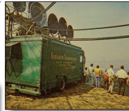
Figure 2.112 At this boat race in the late 1980s, it took a fair-sized truck to house a half dozen microwave transmitters and receivers. Each transmitter would occupy almost a full height rack (almost seven feet tall) and receivers about half a rack. The equipment was quite heavy and produced a large amount of heat.
