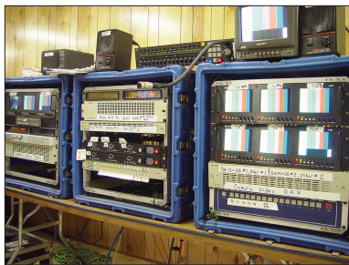
Figure 2.104 The Hi+ effort is often large enough to be a remote in itself. As such, there are companies that specialize in providing those services. These "light cases" are from Broadcast Sports Television (BST). Video from the "catcher" microwave receivers is fed into this office trailer where it can be monitored and distributed to the production trucks.
